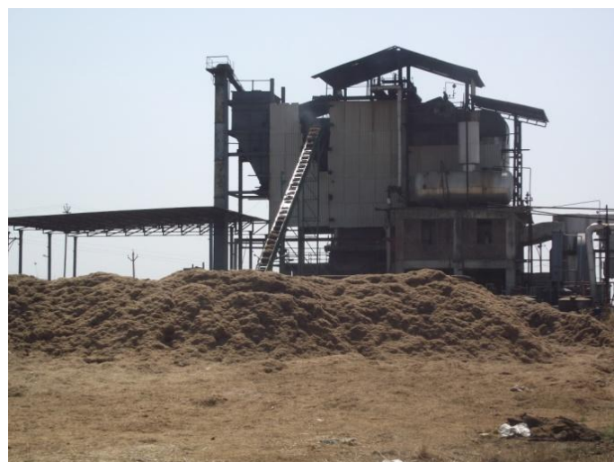
Boilers using biomass at Narmada Solvex
